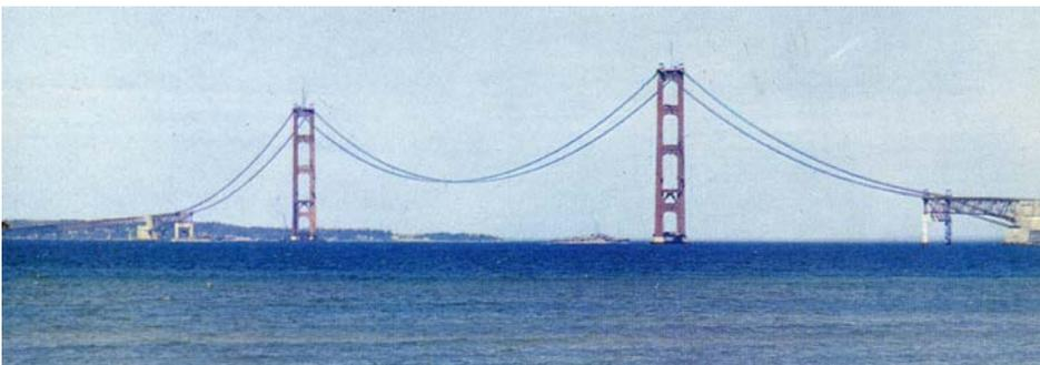
Left - The Mackinac Bridge under construction as it appeared over 50 years ago. Construction first began in May 1954. The two support towers are 752 feet high, 552 feet of which are above water. Notice the roadway had not yet been constructed when this photo was taken.
